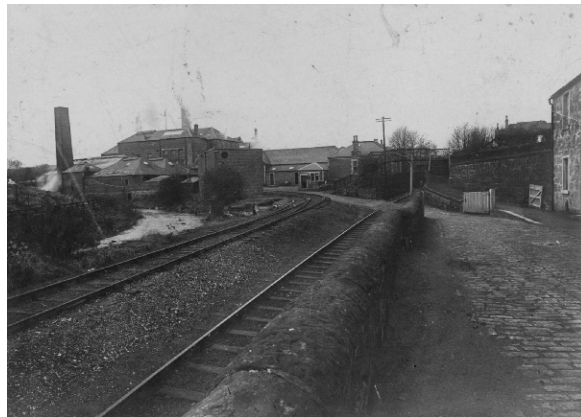
The railway spur line at the paper mill. The former track bed on the right now forms the start of the West Highland Way which passes through the cutting under the location of the former foot-bridge on the right
